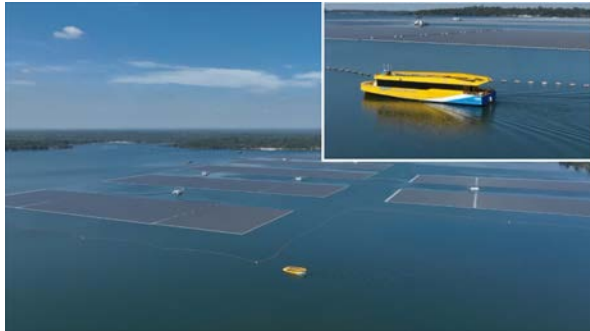
Figure 15 Electric-powered workboat at the hydro-floating solar hybrid system
