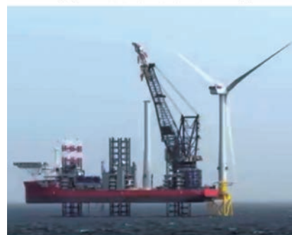
(b) Wind turbine installation
