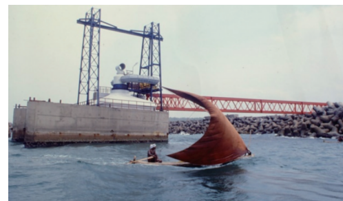
Figure 11 OWC-based wave energy plant (Hodgins et al., 2008)
