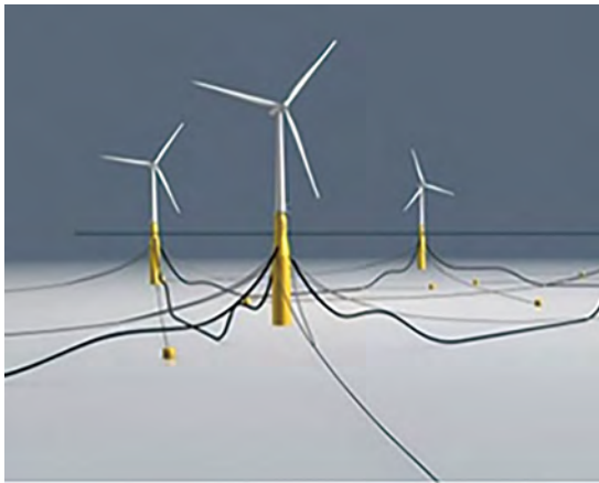
Figure 1 World's first floating wind turbine, Hywind (Madslie, 2009)
