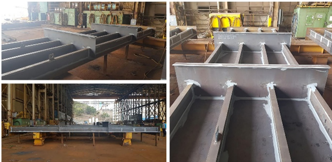
Figure 6 The plate panel after completing of fabrication in the shipyard
