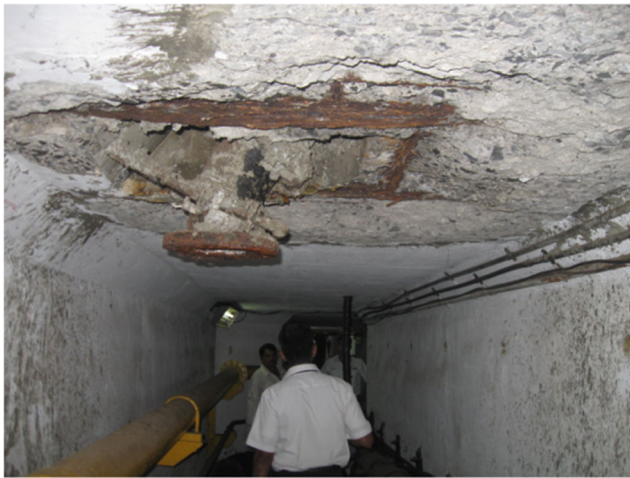
Fig. 1 Visual inspection at a colossal marine concrete structure
