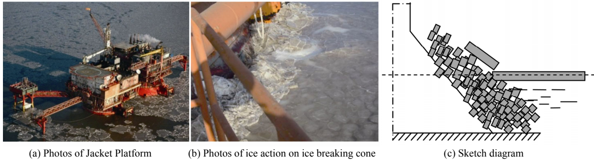
Fig. 3 Broken ice pile-up on JZ9-3 Caisson
