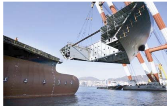
Fig.1 The block erection using crane vessel
