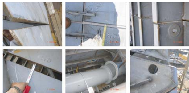
Fig.2 The misalignment problems of adjacent blocks in the erection stage
