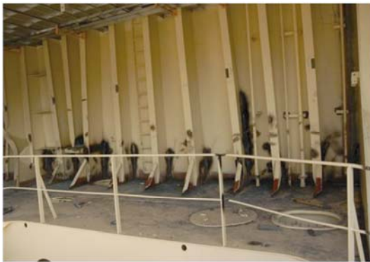
Fig.4 Cutting the inner parts for closing a gap between upper block and bottom block
