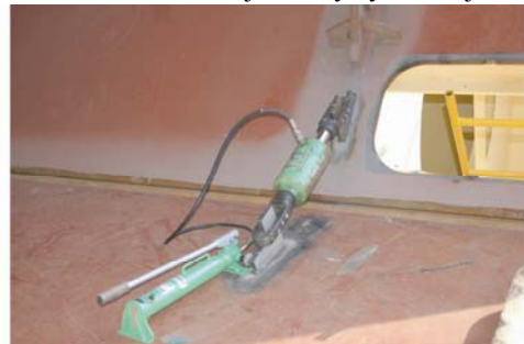
Fig.16 The hydraulic jockey was installed on the block to adjust the position of block in detail
